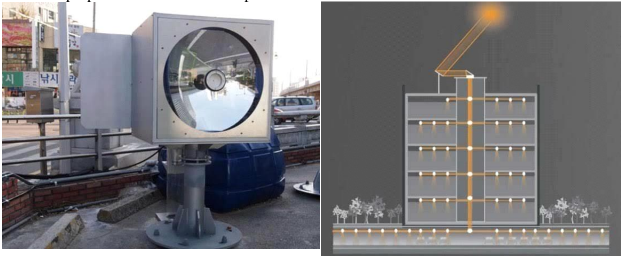
Figure 2.3: Sun Portal, use of Fiber Cable
